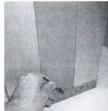
6. Replace single retaining screw.
